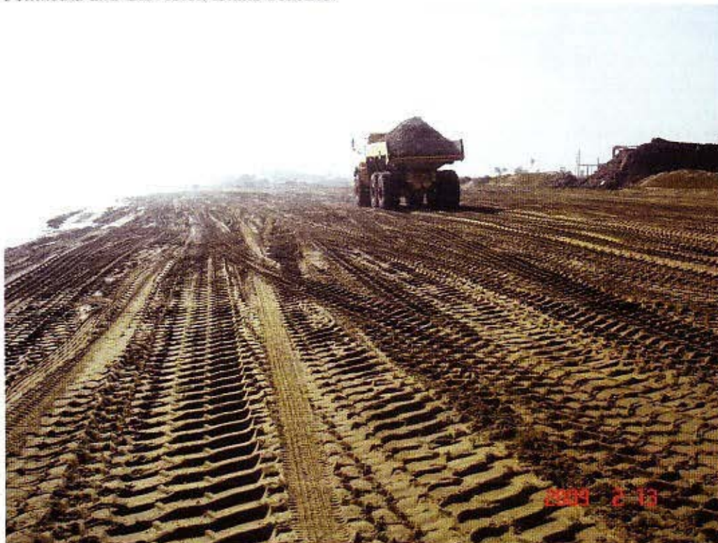
Figure 12. Bolivar Peninsula beach exhibiting highly compacted sand substrate as a result of heavy equipment used in renourishment activities.
