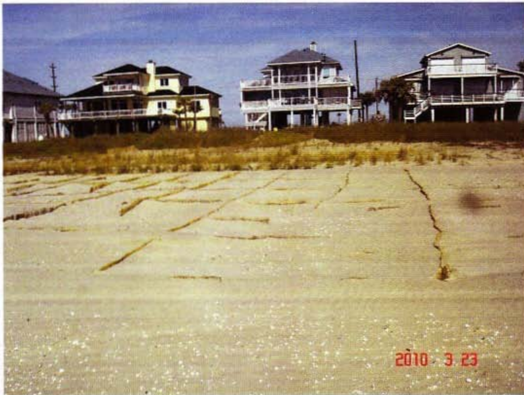
Figure 29. Assortment of sand accreting features including perpendicular and parallel fences bordering rows of planted vegetation on West Galveston Island.
