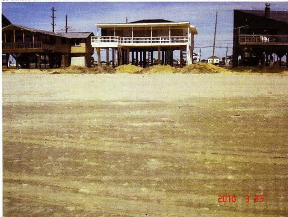
Figure 14. West Galveston Island site where non-sand substrate(s) is used as a dune renourishment initiative.
