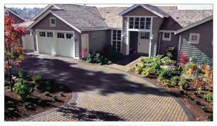
Figure 4-4: Driveway constructed of permeable pavers. (Photo courtesy of Mutual Materials)
