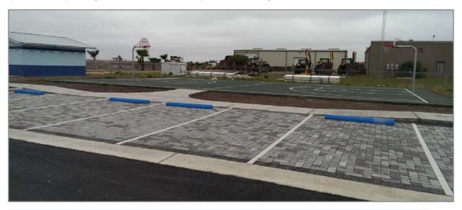
Figure 5-5: Permeable pavers in parking stall of Cascade Park parking lot in Cameron County.
