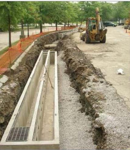
Figure 6-3: Adding a sand filter to treat parking lot runoff
