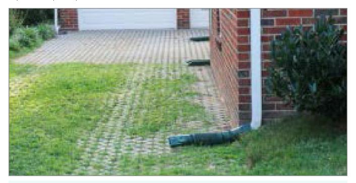
**Figure 2-5:** Downspouts directed to permeable pavement on driveway. (Photo courtesy of Montgomery County, Maryland)
