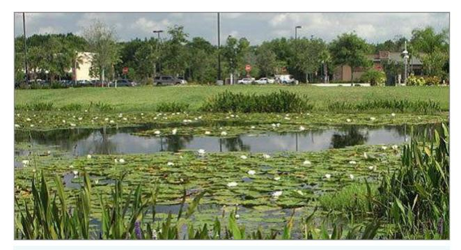
**Figure 5-8:** Picture of an enhanced detention wet pond. (Photo courtesy of Houston-Galveston Area Council)
