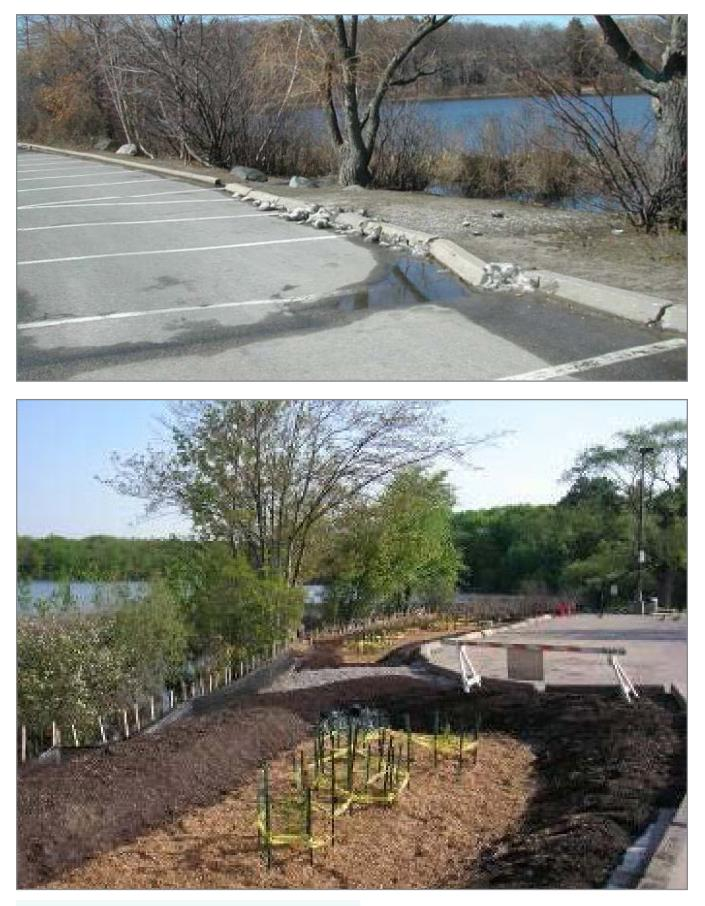
Figure 6-2: Adding a bioswale at edge of a parking lot
