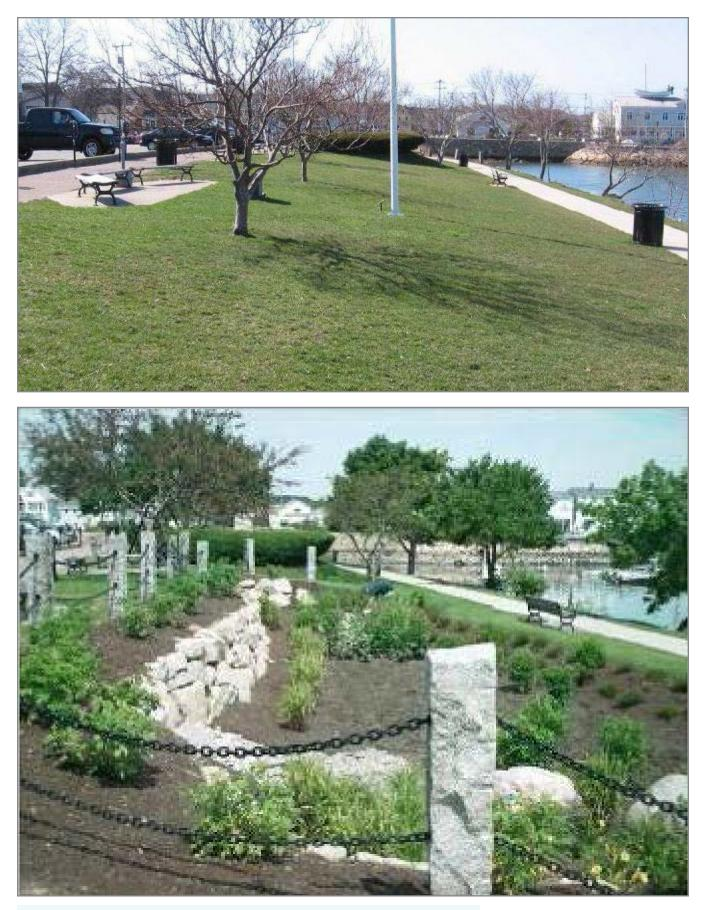
**Figure 6-1:** Adding a Bioretention basin (rain garden) in a municipal park
