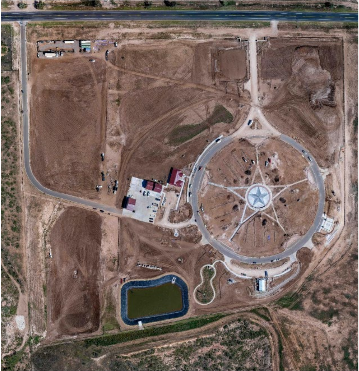
Drone view of project
