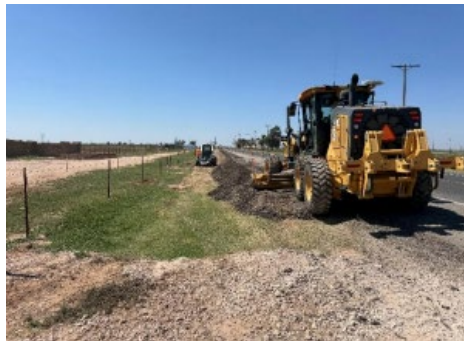
TXDOT working on deceleration lane on 50 th St
