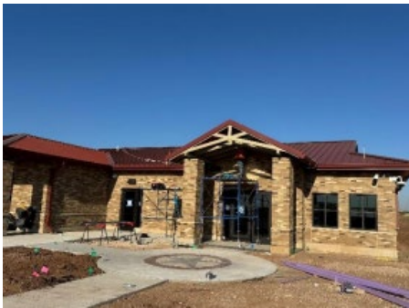
Work continues on the Administration Building
