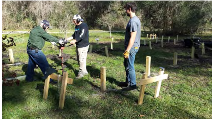
(L) TCWP staff stake the locations of the nursery tanks. (R ) Holes are dug by auger and 4' posts of 4x4 are placed.
