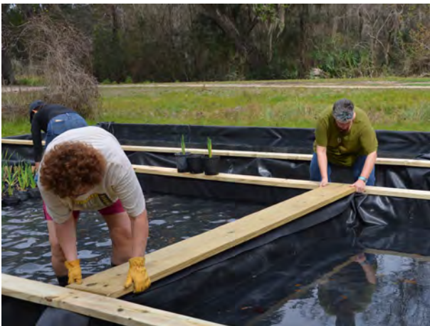
(L) The top coping is installed over the pondliners. Photo: Pete Romfh (R ) Coping placement continues .
