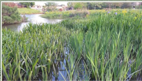
One stormwater wetland example is at Mason Park in Houston, which filters runoff from a nearby neighborhood before it enters Brays Bayou.
