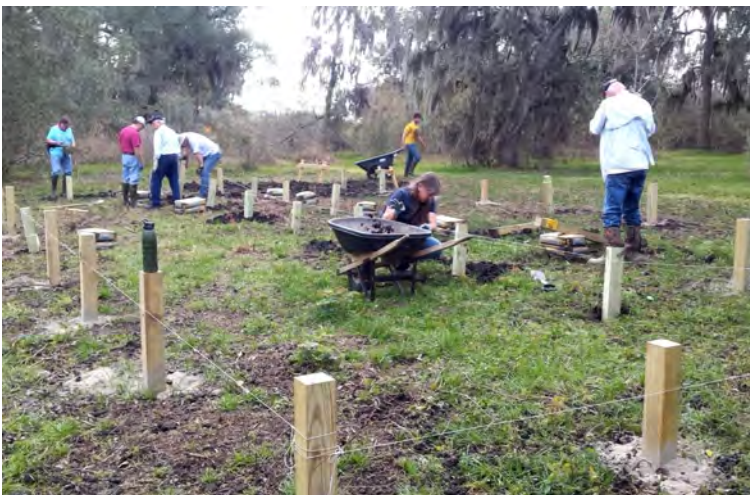
(L) volunteers complete setting of the posts. (R ) Framing of the tanks begins. Photo: Dave Brandes
