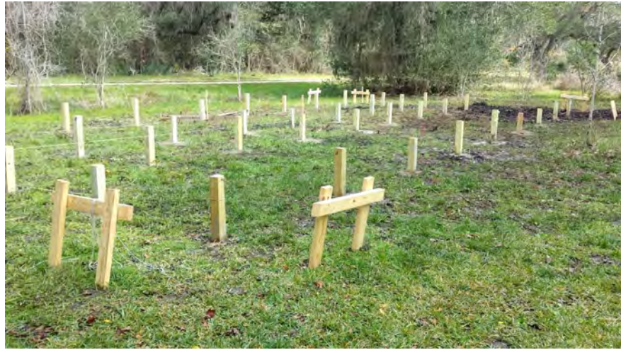
(L) Posts are anchored in concrete. Photo: Pete Romfh (R ) The site with posts partially set.
