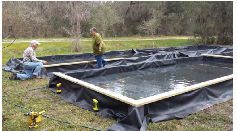
(L) The top coping is installed over the pondliners. Photo: Pete Romfh (R ) Coping placement continues .
