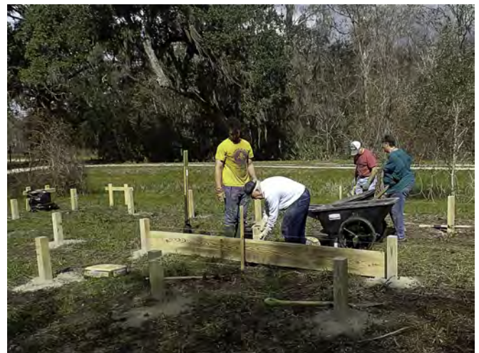
(L) volunteers complete setting of the posts. (R ) Framing of the tanks begins. Photo: Dave Brandes
