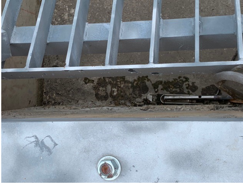
Figure 15. Outflow structure at PTWB.
