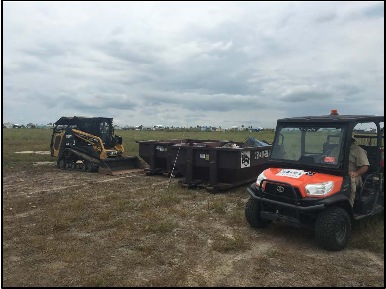
Contractor with some equipment used in the debris removal effort
