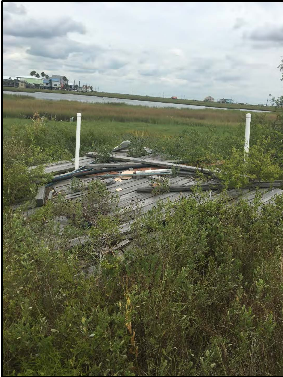
Section of a deck resting on top of a boat trailer. Items were removed as part of the debris removal effort
