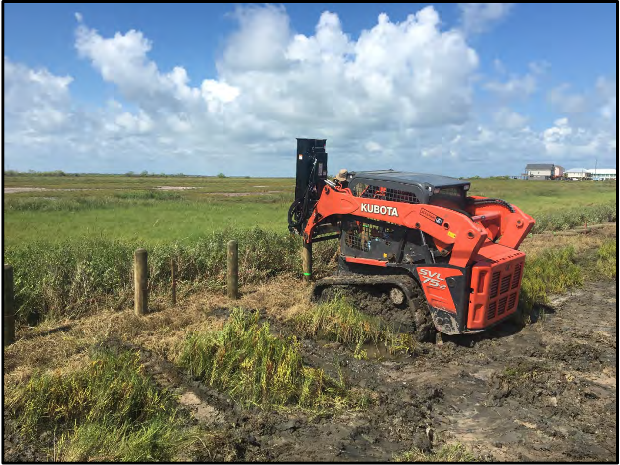
Copano Bay Excavation Using Hydraulic hammer to install bollards
