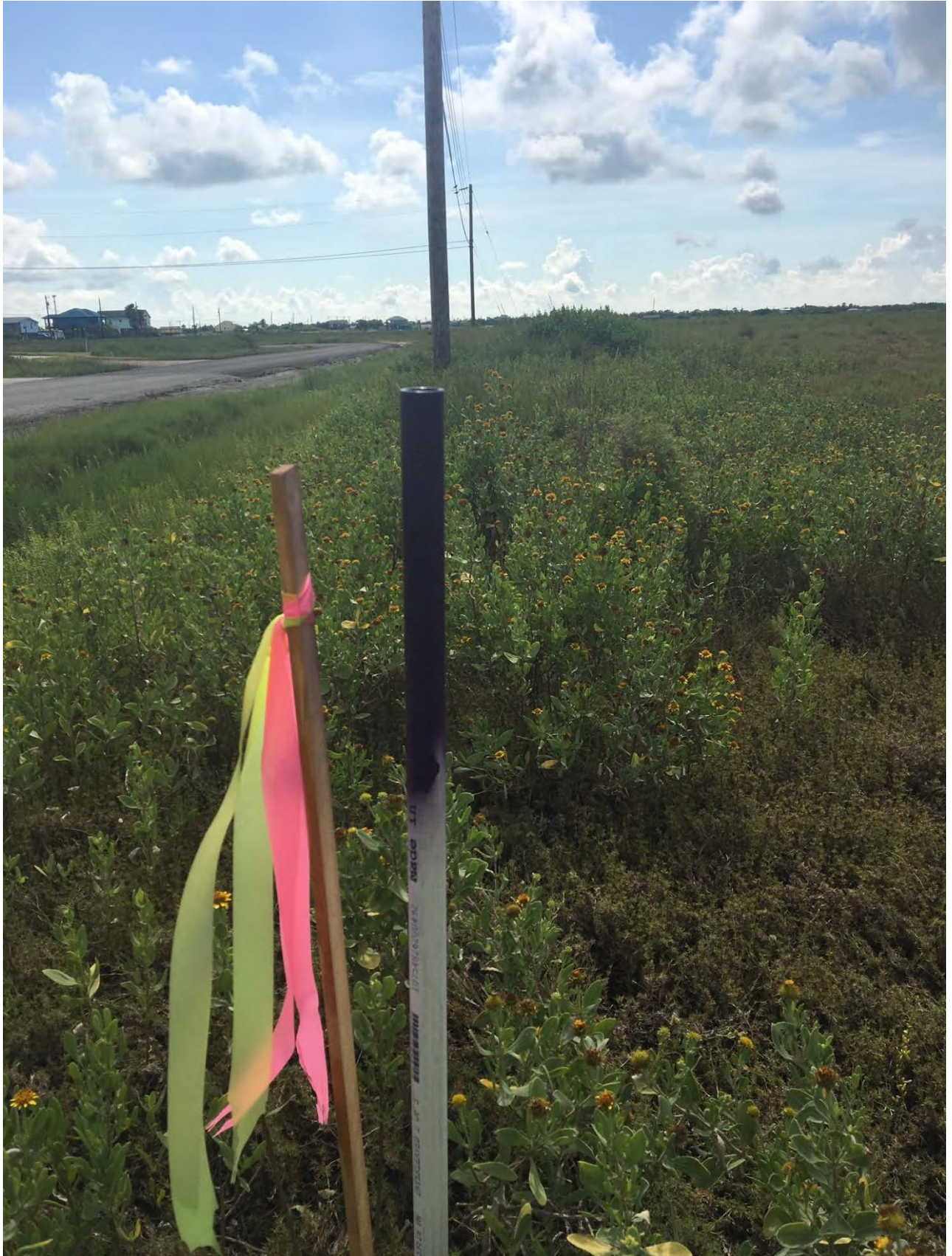
Property boundary marked by Surveyor. PVC marker installed to delineate future bollard line.
