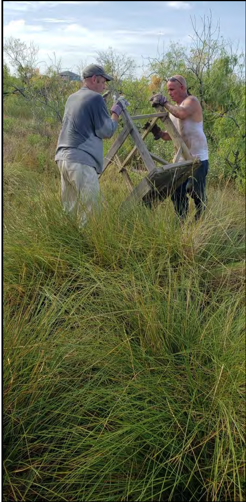
Laborers working in Tract A removing debris
