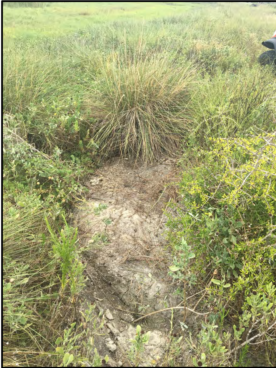
Bare ground in a vegetated high marsh area. Section of roof was covering the vegetation
