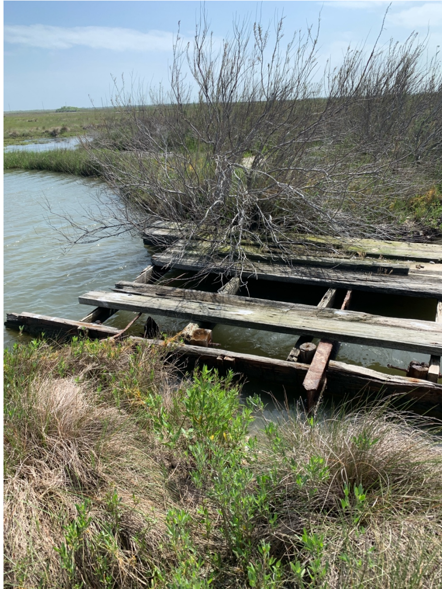
Fig. 29. An old, damaged bridge on Chinquapin Bayou.
