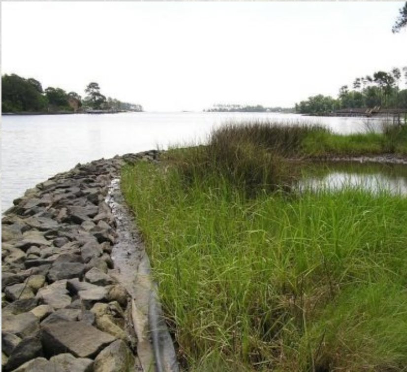
Marsh Toe Revetment [Center for Coastal Resources Management]
