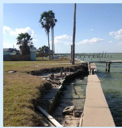
Bulkhead Failure Leads to Erosion and Land Loss Photo: Texas General Land Office
