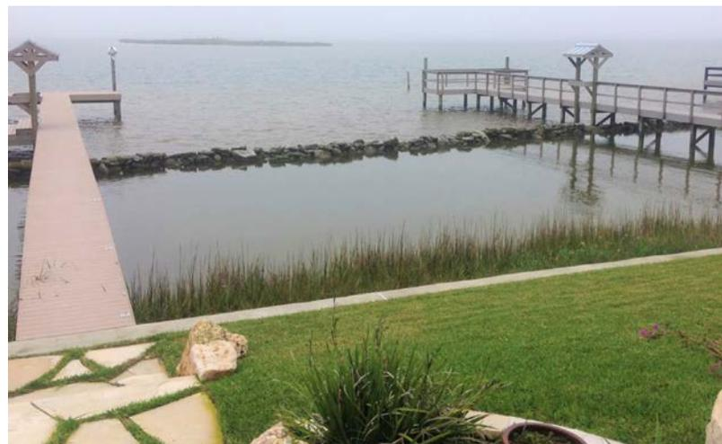
*Rock Rubble Breakwaters Protecting Area of Planted Seagrass (Under the Water) and Cordgrass Along the Bulkhead.
