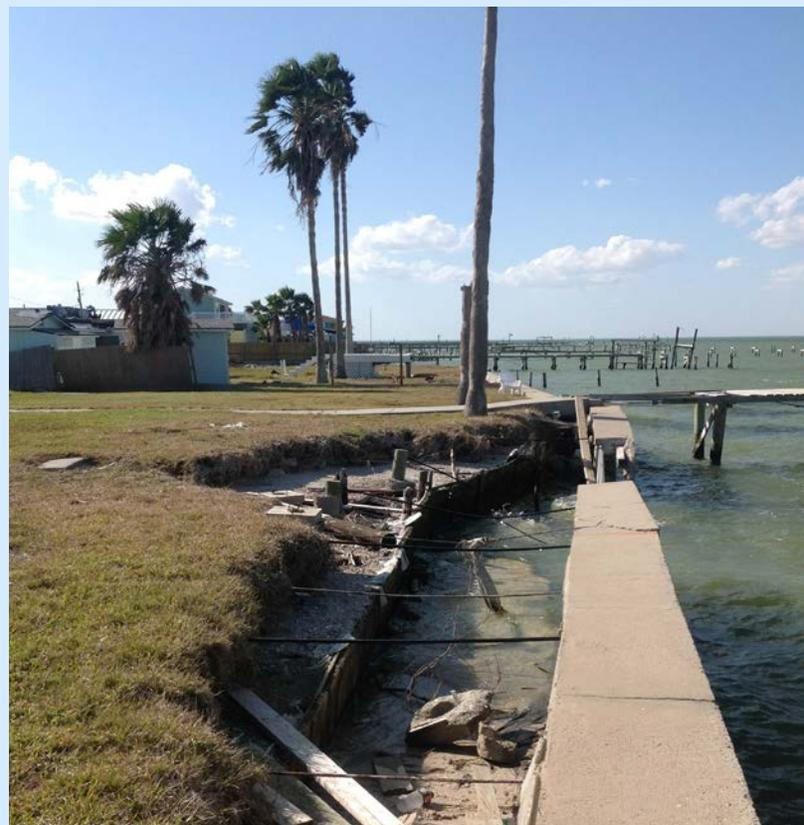
*Bulkhead Failure Leads to Erosion and Land Loss
