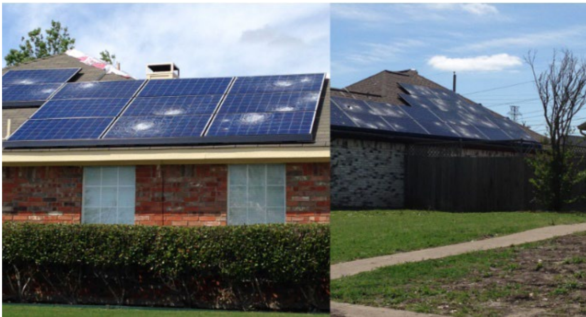
Figure 3-46: Hail damage to residential solar panels. 216
