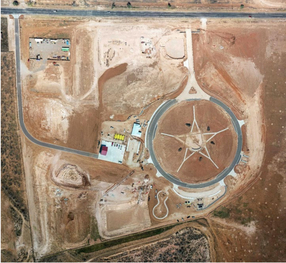
Drone view of project
