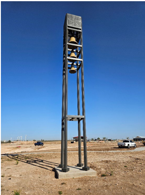
The bell tower installed
