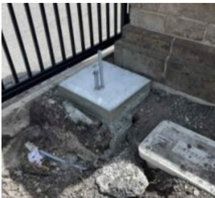
Automatic main gate closure system installation
