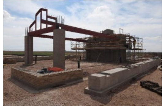
Rebuilding of the Committal Shelter
