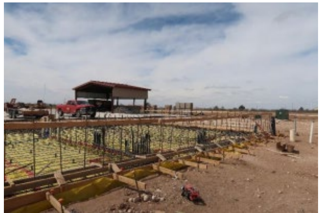
Pouring of Maintenance building foundation
