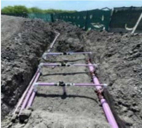
Irrigation line installation
