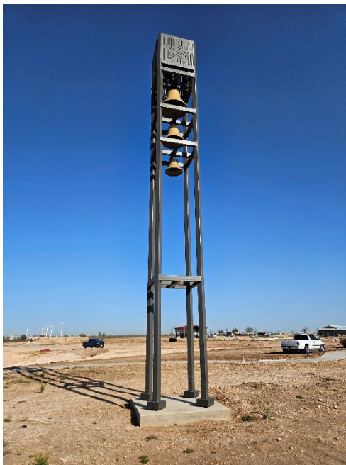
The bell tower installed
