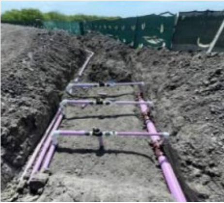
Irrigation line installation
