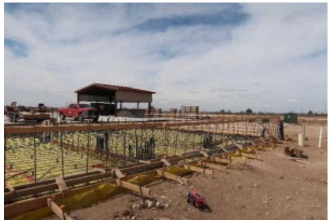
Pouring of Maintenance building foundation
