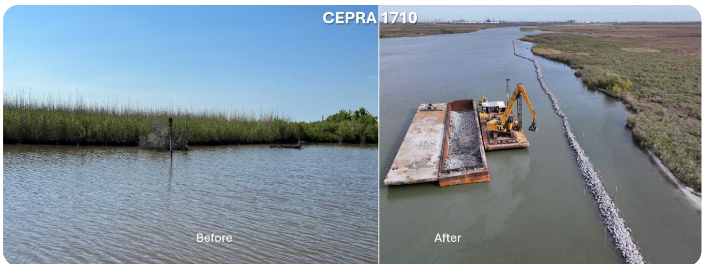
Figure 23. Breakwater along JD Murphree WMA.
