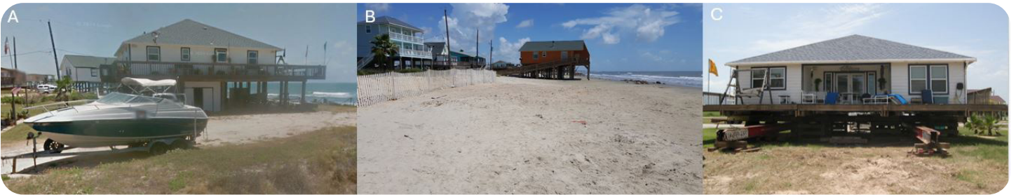
Figure 5. CEPRA Structure Relocation at Surfside. A. The structure before removal on the public beach easement. B. The pad-site after the structure is removed. C. The structure moved to a new location.
