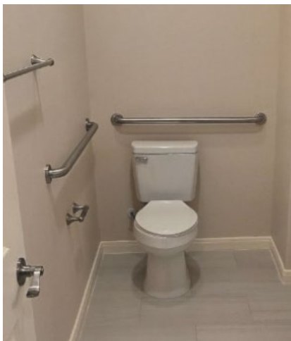
Grab Bars Around Toilet
