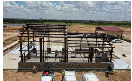
Brick work on Maintenance Building
