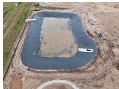
Liner installation at the irrigation pond
