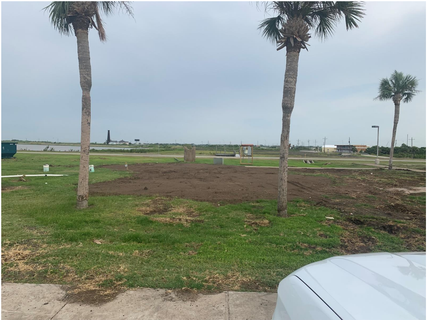
Site after Demolition
