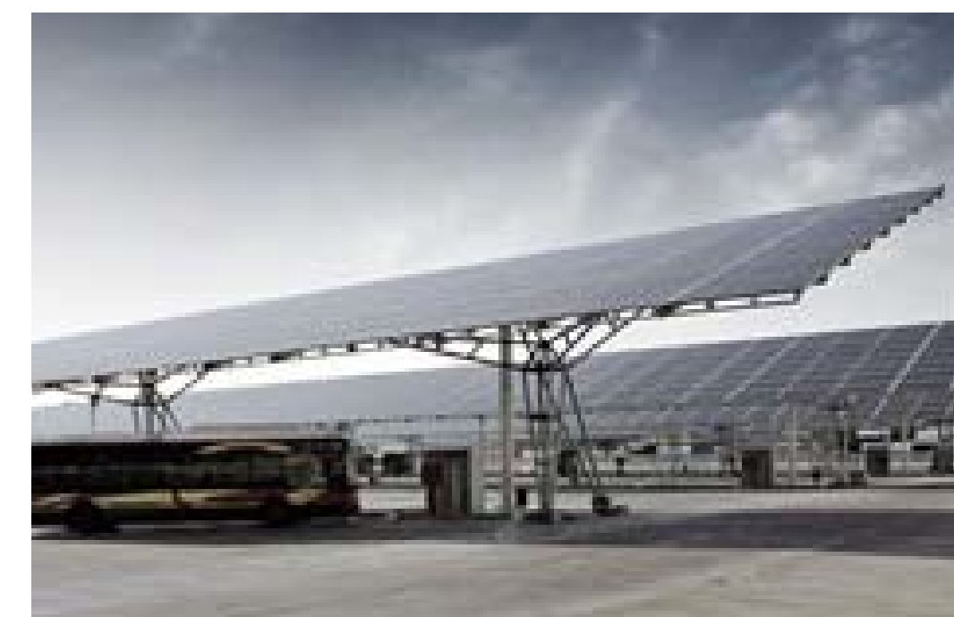
Solar Panel Covered Walkway
