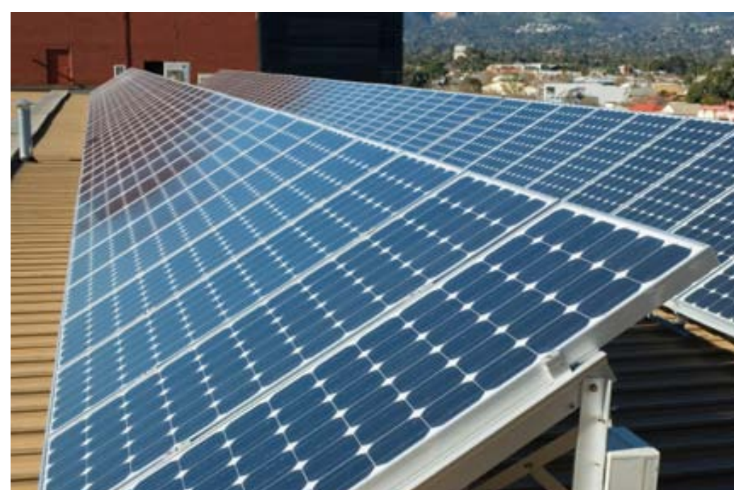
Static Photovoltaic Array
