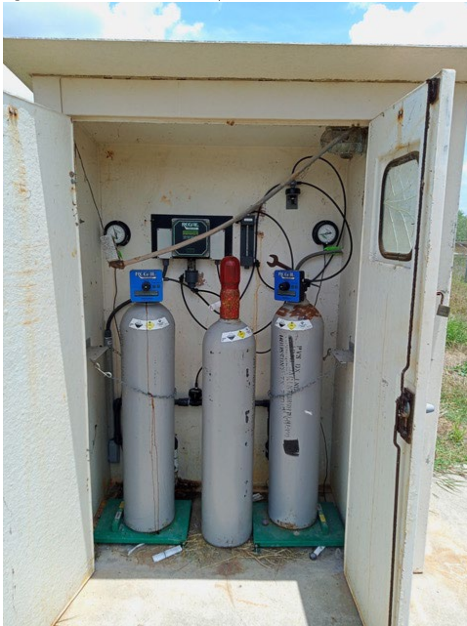
Figure 6: Chlorination chamber replacement the Driscoll WWTP
