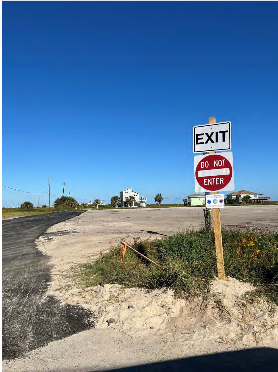
Photo 19: Exit Signage View to East
