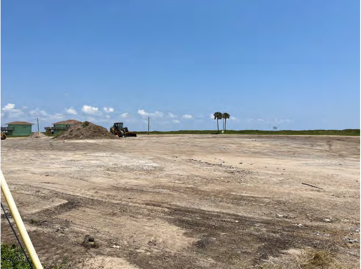
Photo 5: Grading of Site View to South
