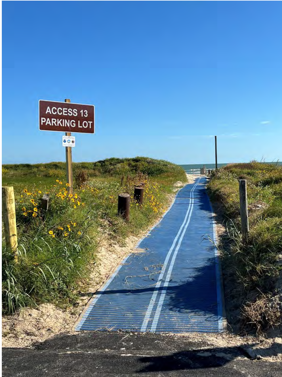
Photo 18: Finished Pedestrian Beach Access with Signage View to South
