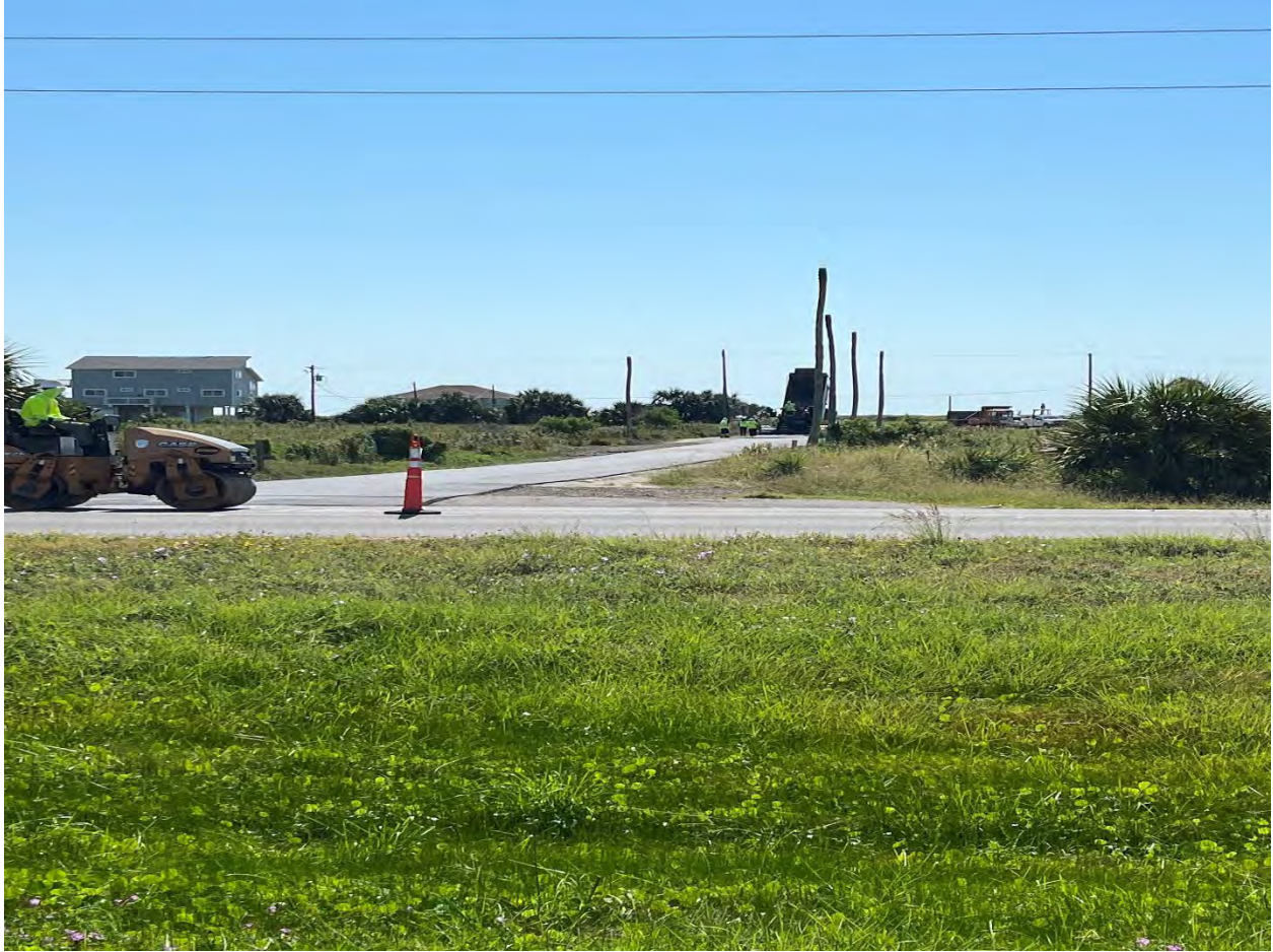
Photo 9: Laying of Asphalt on Access Road from FM 3005 to Parking Lot
