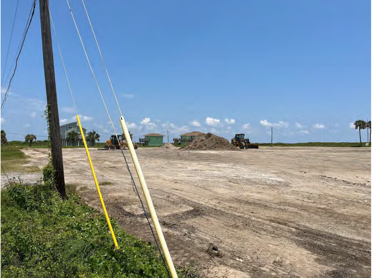
Photo 6: Grading of Site View to East
