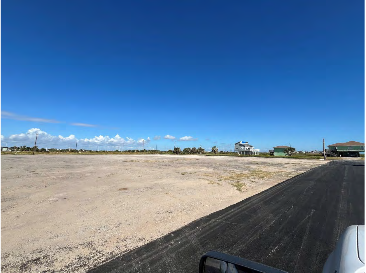
Photo 13: Finished Parking Lot and Access Road View to East
