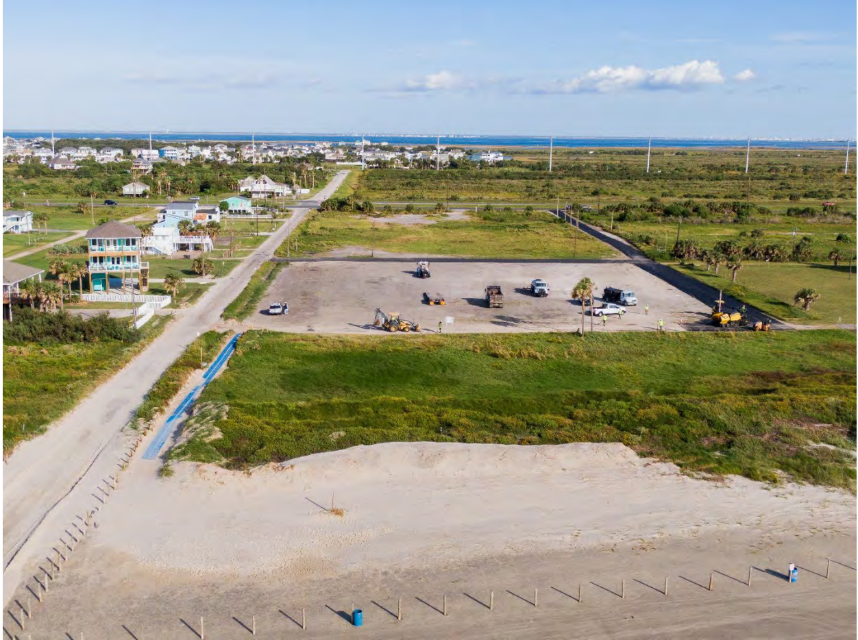
Photo 11: Drone Photo of Site Work
