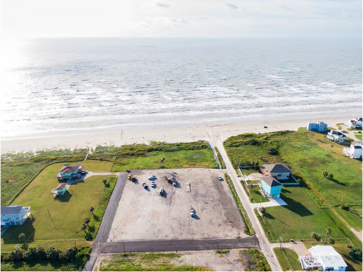
Photo 10: Drone Photo of Site Work
