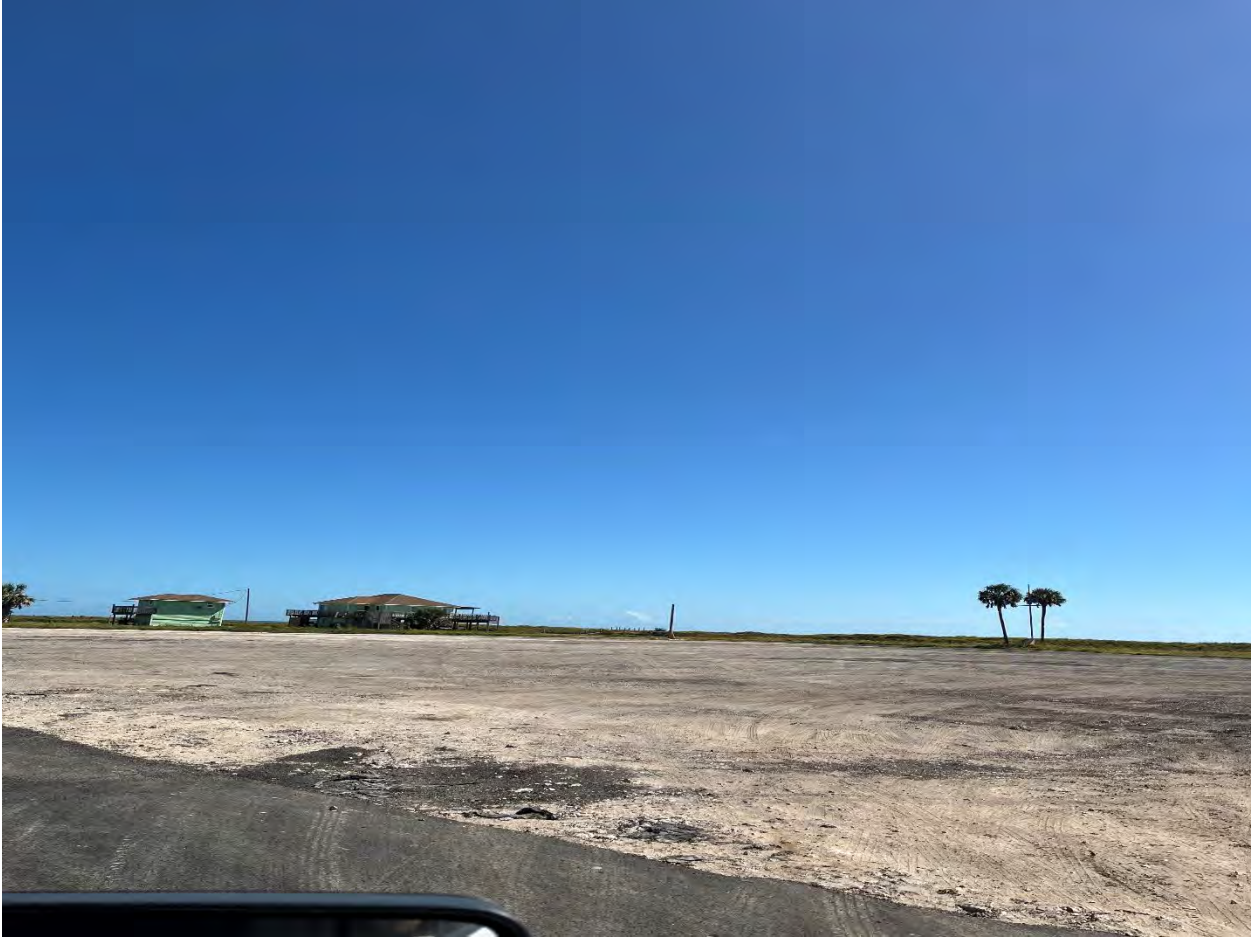
Photo 14: Finished Parking Lot View to South
