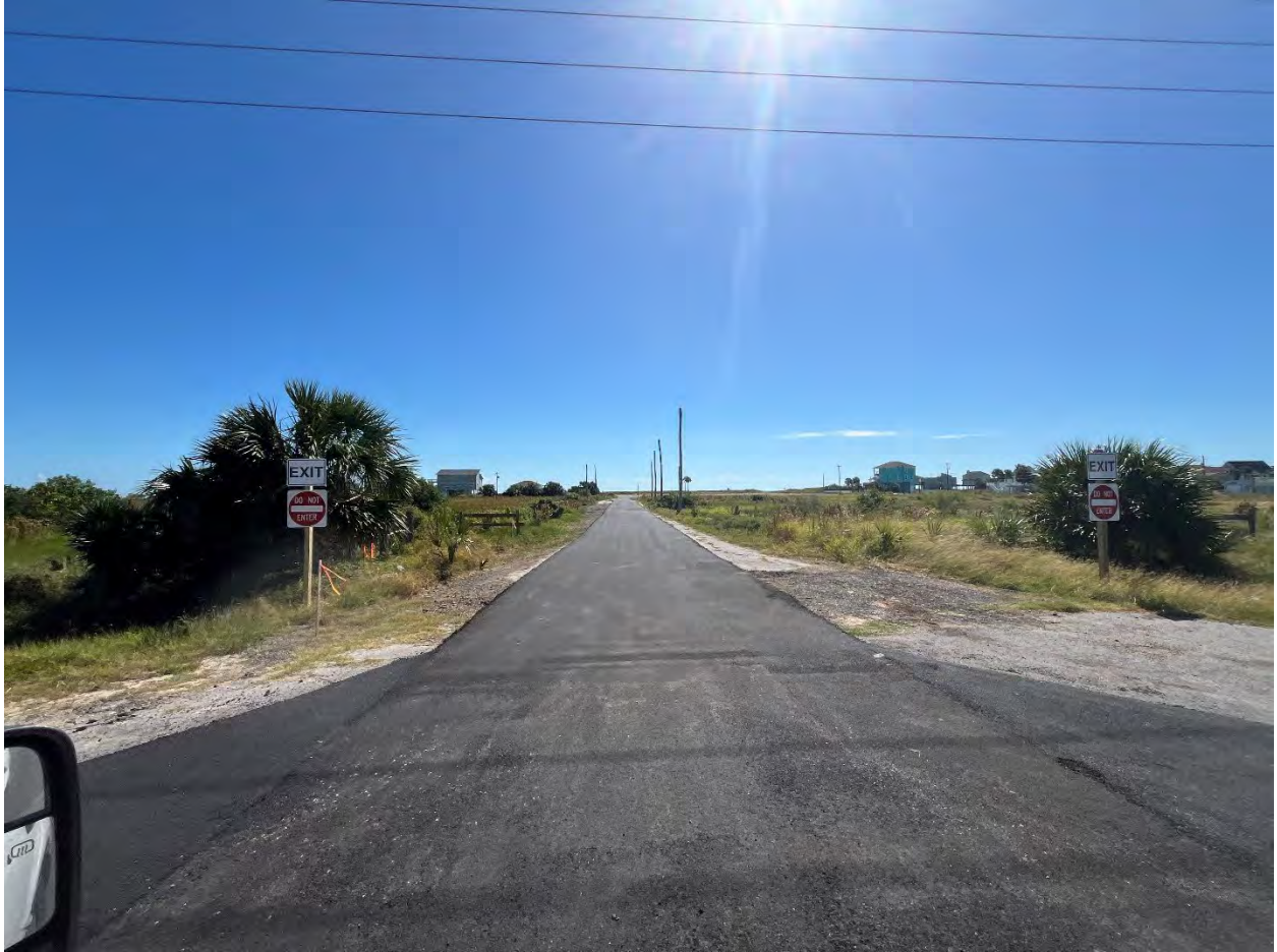
Photo 16: Finished Access Road from FM 3005 to Parking Lot with Signs View to South
