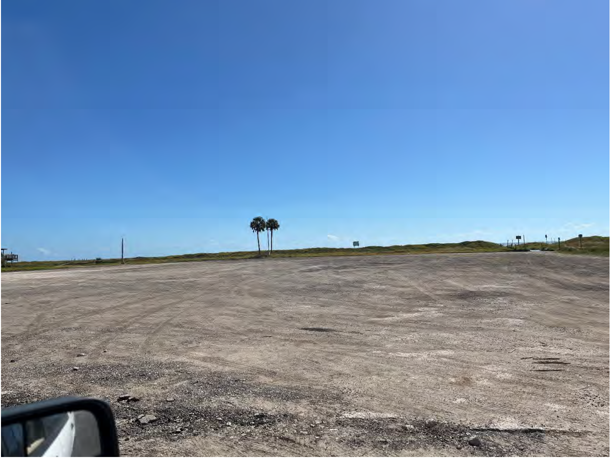
Photo 15: Finished Parking Lot View to South
