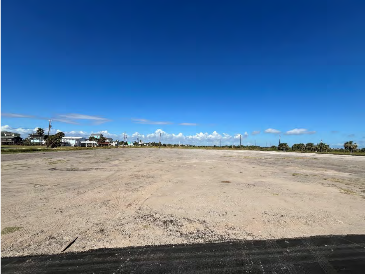
Photo 12: Finished Parking Lot View to North
