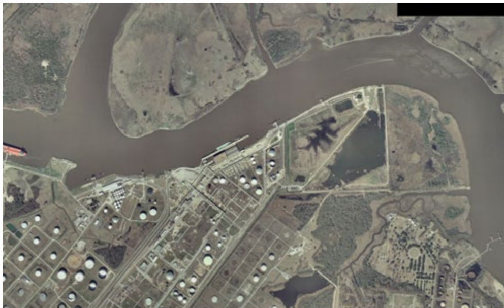
Picture 1: Chevron Beaumont Terminal in Beaumont, TX
