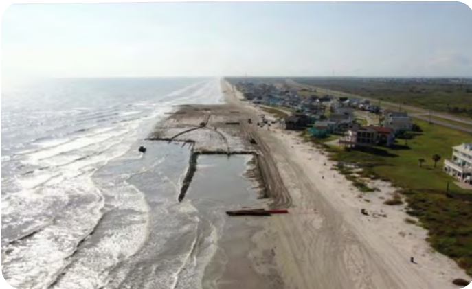
The GLO, the City of Galveston, and the Galveston Park Board partnered with the US Army Corps of Engineers to oversee the placement of Beneficial Use of Dredge Material beach quality sand.
