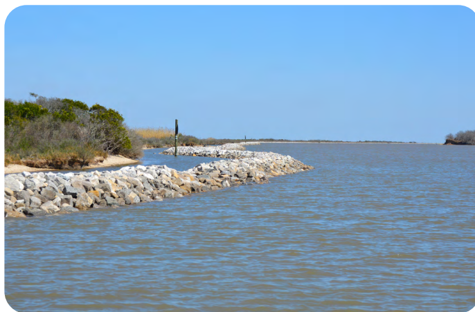
Newly constructed breakwaters completed in March 2026 protect the Mad Island WMA property.
