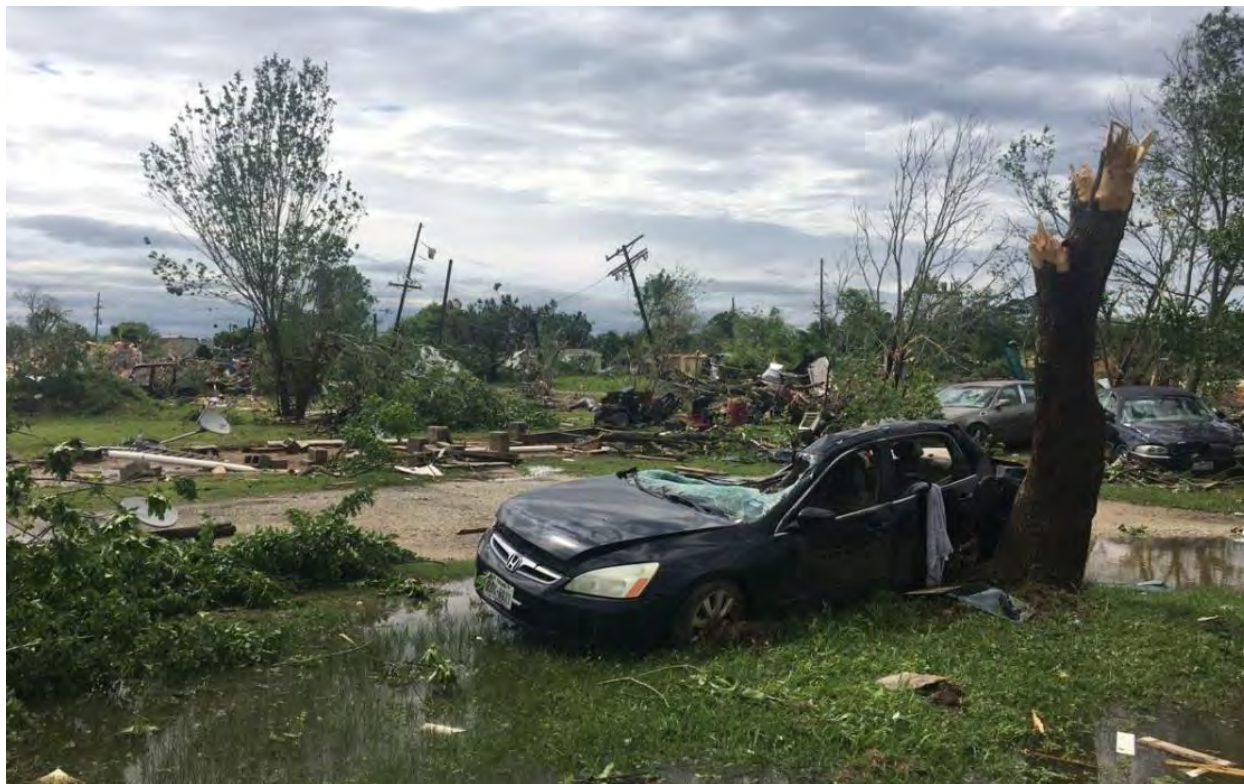
Figure 3-50: Tornado damage in Franklin, April 2019. 242
