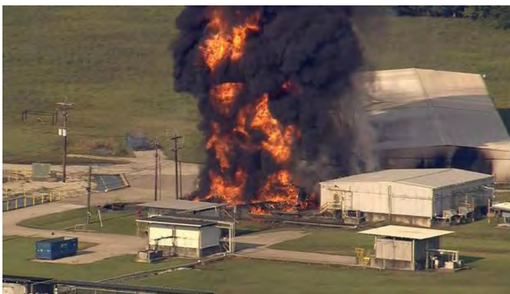
Figure 3-67: Arkema chemical plant explosion in Crosby in 2017. 404
