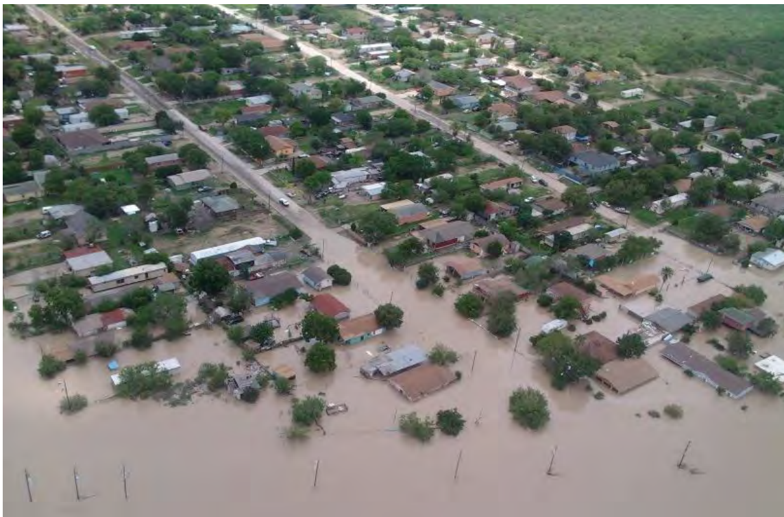
Figure 3-36: Laredo, Texas, during 2010 Flooding. 144
